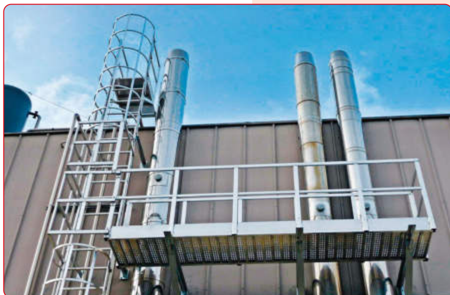
• Example of using an aluminium walkway
